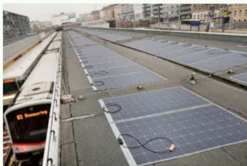
Adhesive PV films on an underground station
