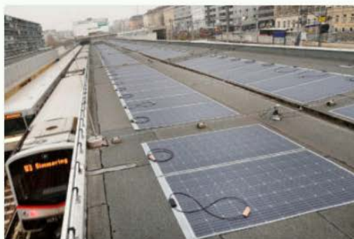
Adhesive PV films on an underground station
