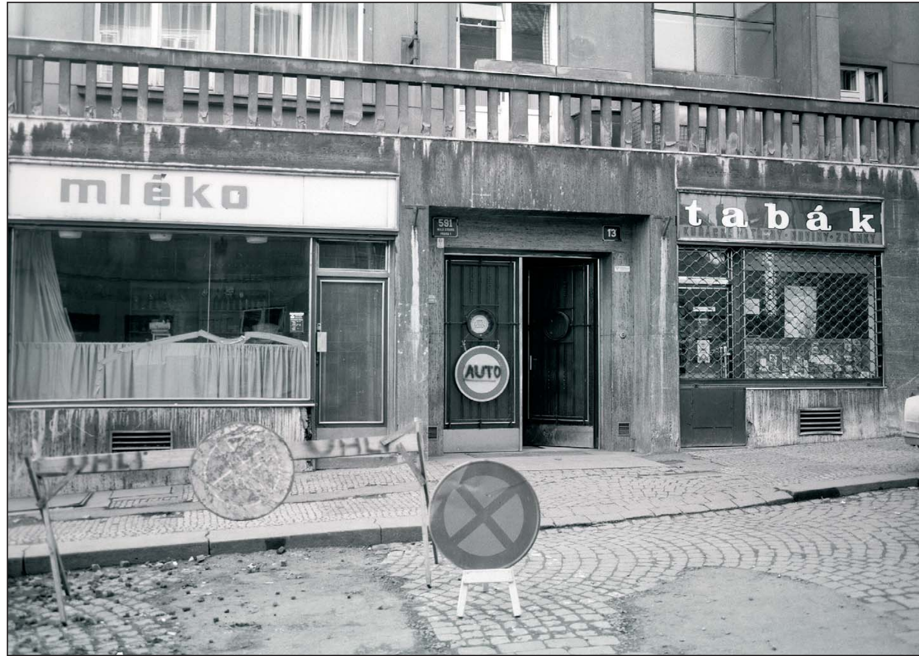
Vlašská ulice, Malá Strana, Praha 1 Vlašská Street, Malá Strana, Prague 1
