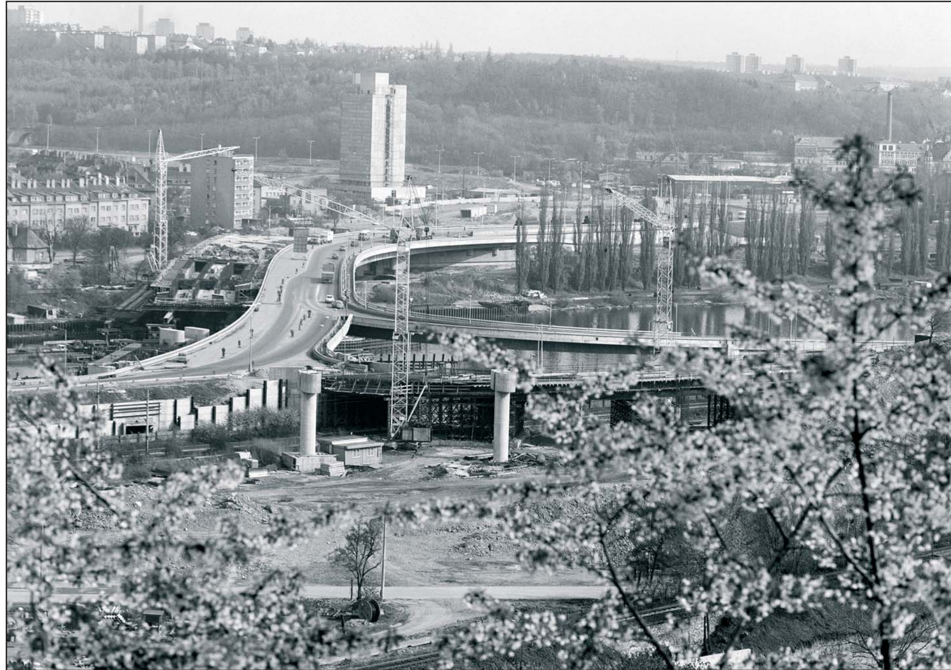
Barrandovský most, spojnice Braník a Hlubočep, Praha 4 a Praha 5 Barrandov Bridge, linking Braník and Hlubočepy, Prague 4 and Prague 5
